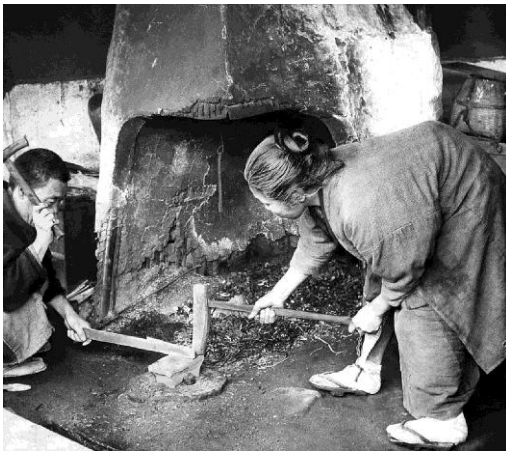
A blacksmith and his wife forge a blade, ca. 1904-05. Hand-tinted glass lantern slide printed from a half-stereoview negative. (Courtesy of Okinawa Soba)
